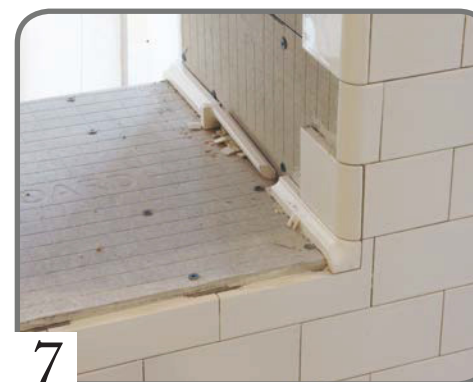
4 Tip: Soaking the tiles in clean water will help give an installer additional time when setting tiles. This will allow the installer to adjust coursing or individual tiles as necessary and flexibility to beat-in the tiles flat.
